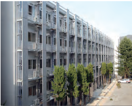
Uji Campus Main Bldg. (M wing)
