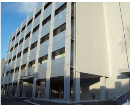
Uji Campus Main Bldg. (W wing)
