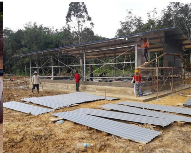
Civil & structural construction
